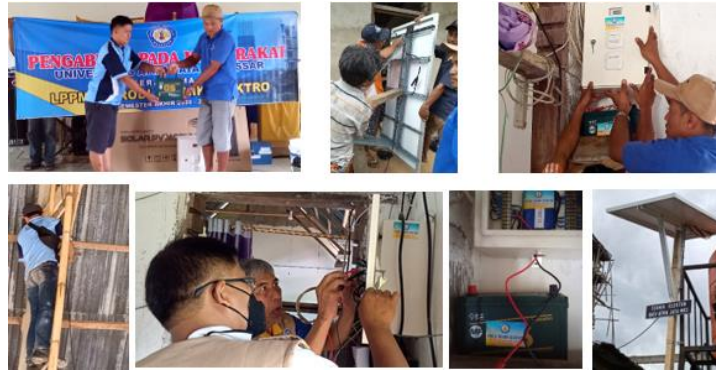
Gambar 8. Kegiatan Instalasi Panel Surya
